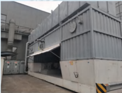
Painting workshop RTO facilities
